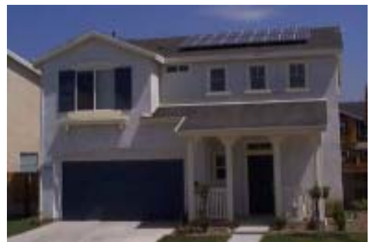
Figure 1 Roof Mounted PV System
