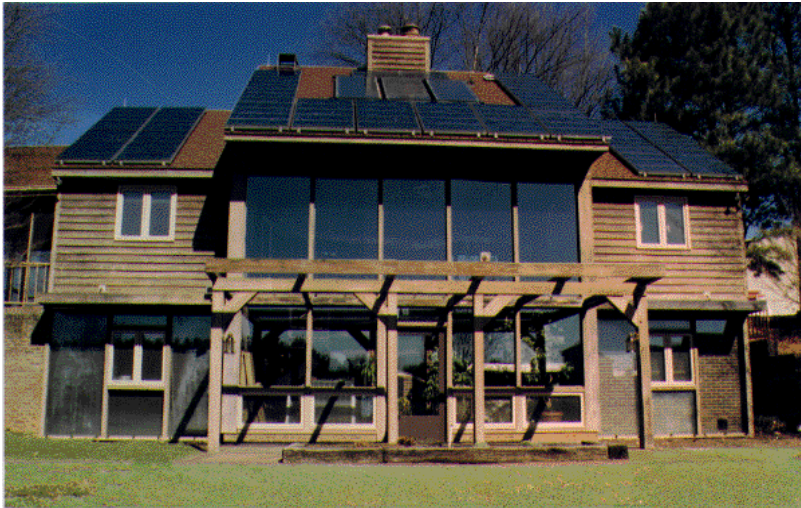
The Solar House at North Carolina State University: A Demonstration Interconnected Residential PV System.
